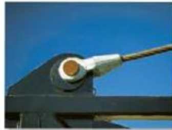
The cable exerts a force on the bracket in the direction of the cable. (1)
